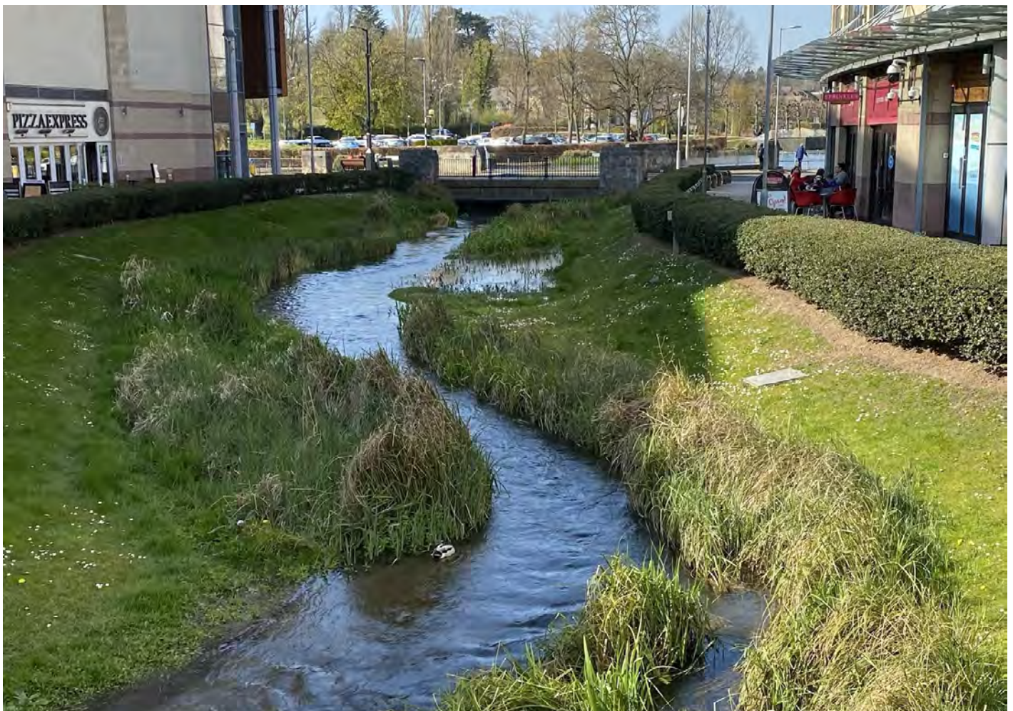
River Gade deculverted and restored as part of Riverside Shopping Centre improvements - Hemel Hempstead
