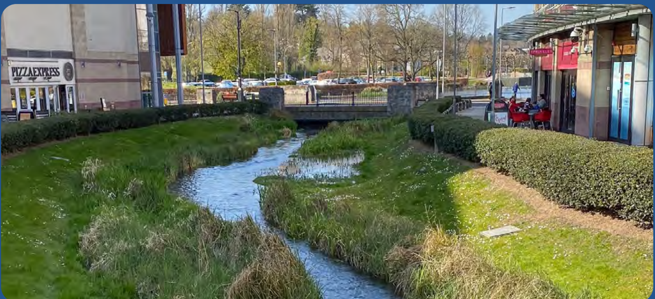
Riverside Hemel, deculverted River Gade
