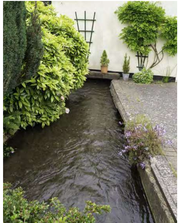
Urban culvert - Hughenden Stream
