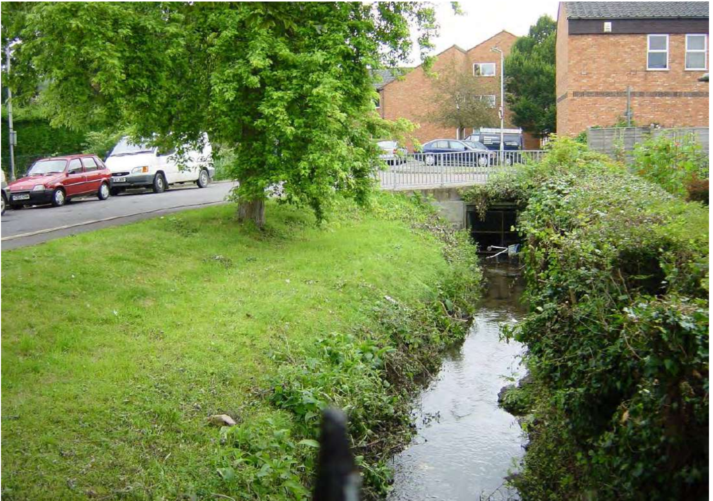
River Bulbourne - Greenfield Road, Berkhamstead
