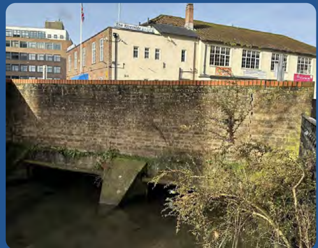
Wye town centre culvert
